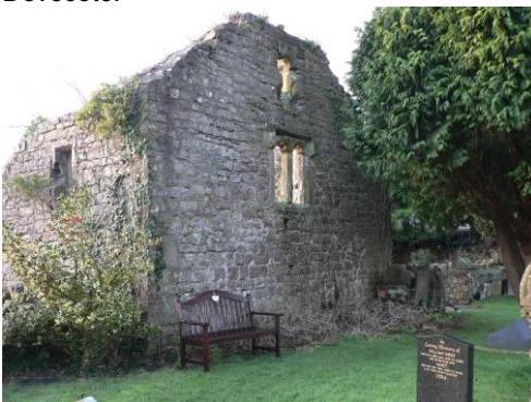
Former Chantry Priest's House.
