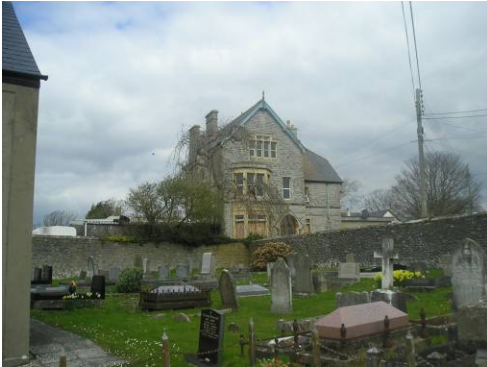
The former Social Club dominates the area from its elevated position above the valley.
