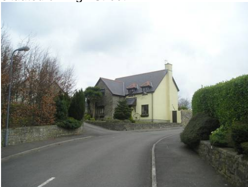
Modern development such as this at Great House Meadows does not enhance the character of the Conservation Area.
