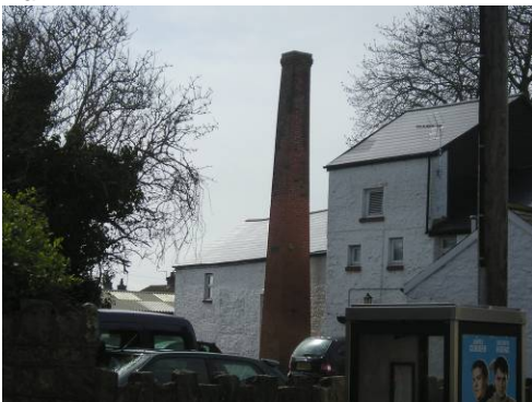
Chimney to former Oast House.
