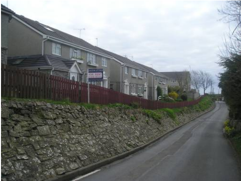
Modern development overshadows the Conservation Area at the south of Colhugh Street.
