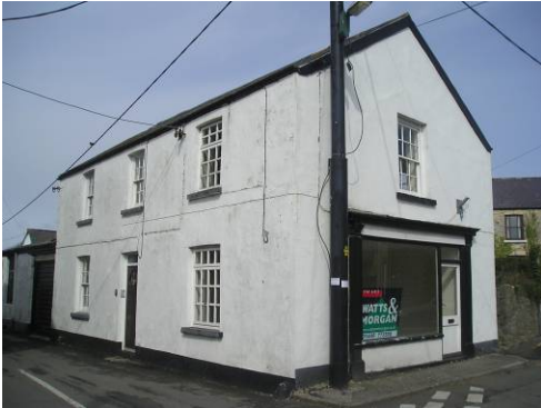
Vacant buildings in the Conservation Area detract from its character.
