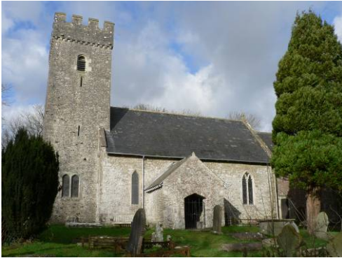
The Parish Church is the principle building in the area.
