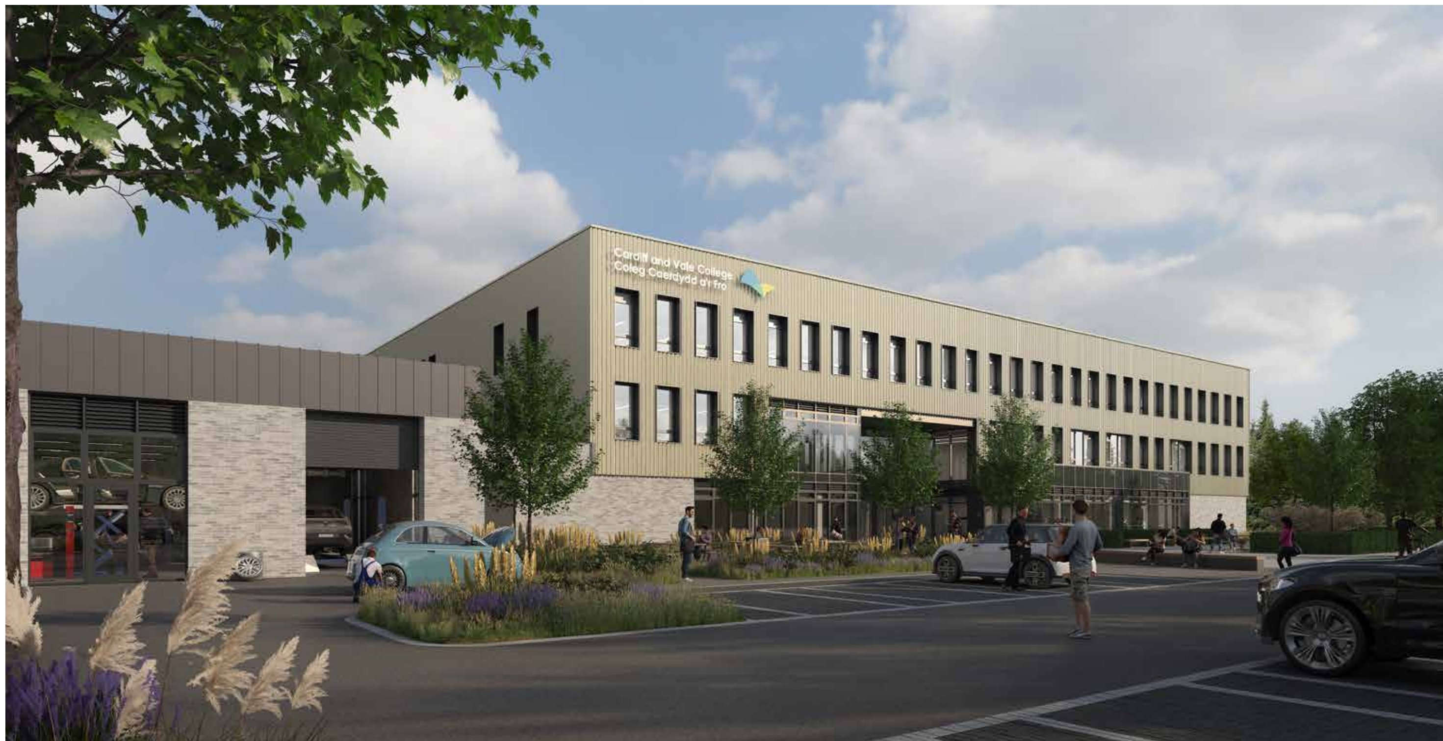
Visual of the rear of the building
