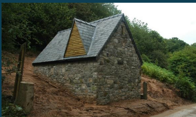
Replacement roost July 2011 (south-western elevation)
