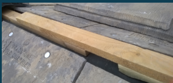
Gaps can be created by using two battens with spaces. In this photo, the ridge roll was omitted (they often contain BRM) and the battens placed directly onto Type 1F 1F bitumen felt. Screws go through the clip/bracket and into the ridge board.
