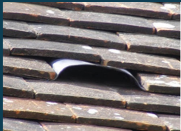
Bat slate in position (neat and unobtrusive).
