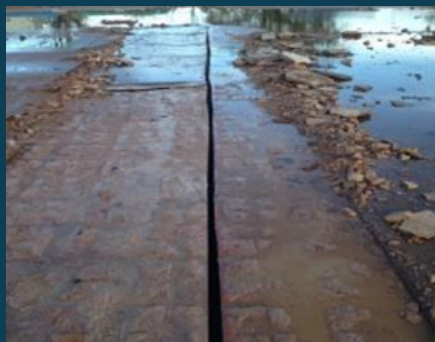
Diamond cut through culvert slab
