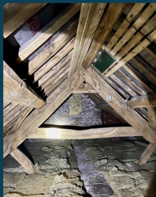
All existing timbers were maintained and droppings retained in the loft space. Interior of roost has additional timber provision and a heating panel (droppings present below this feature).
