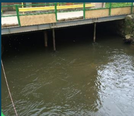
Western end of culvert
