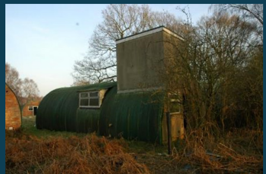
Building prior to start of works
