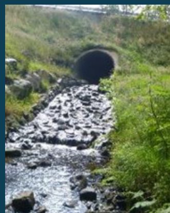
The culvert with stream flowing through
