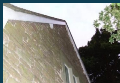
Bat access point at gable apex
