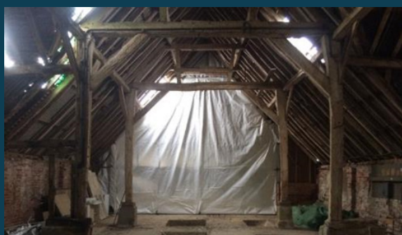
Screening in place
