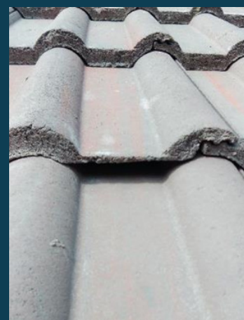
Crevice access created by cutting a notch in the tile to create a gap (20 mm wide and the length of the tile)
