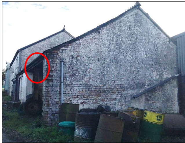
Plate 7: Section C (barn complex) and confirmed pipistrelle species roost, red circle indicates where bats emerged.
