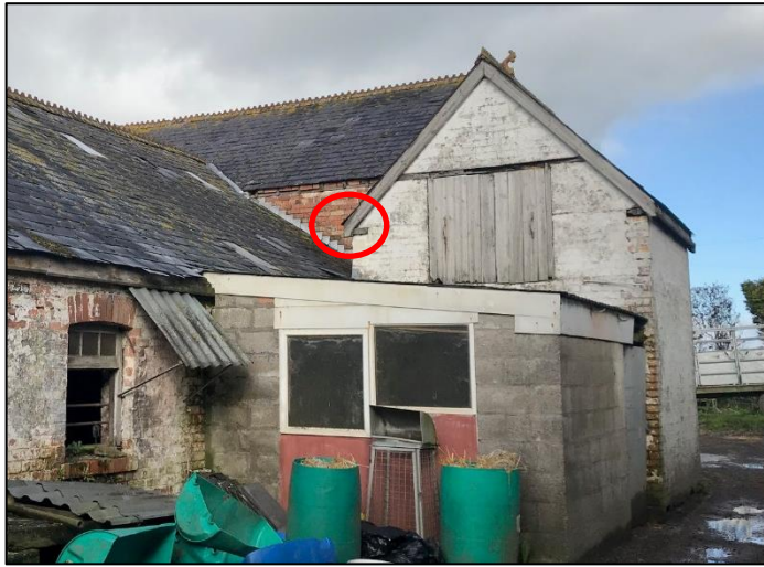
Plate 5: Section A (barn complex) and confirmed soprano pipistrelle roost, red circle indicates where bats emerged.
