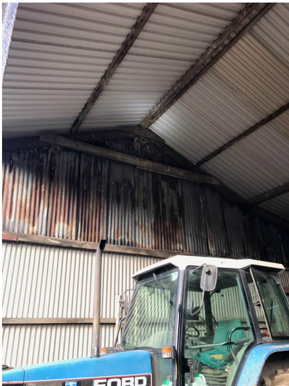
Figure 2 Internal structure of Barn D
