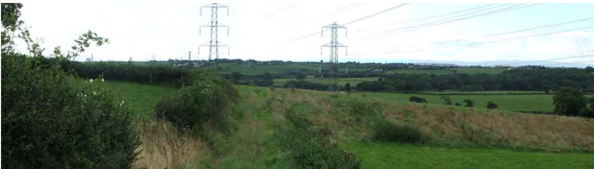
Lower Thaw Valley looking south towards St Athan
