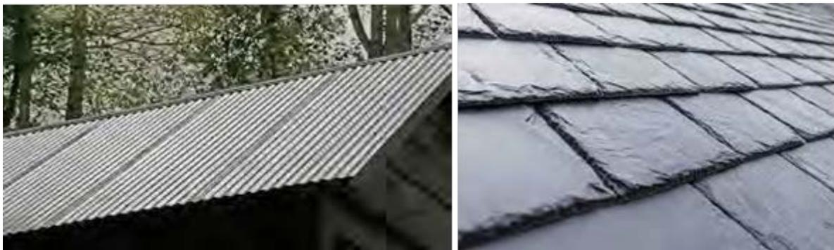
9.5.3. Verges and eaves details are often overlooked when converting a rural building. Verges often comprise simple slate on stonework with a maximum 40-50 millimetre overhang. Modern bargeboards / soffit details with overhangs are not appropriate. Careful consideration should be given to an appropriate eaves detail which replicates the original character of the building.
