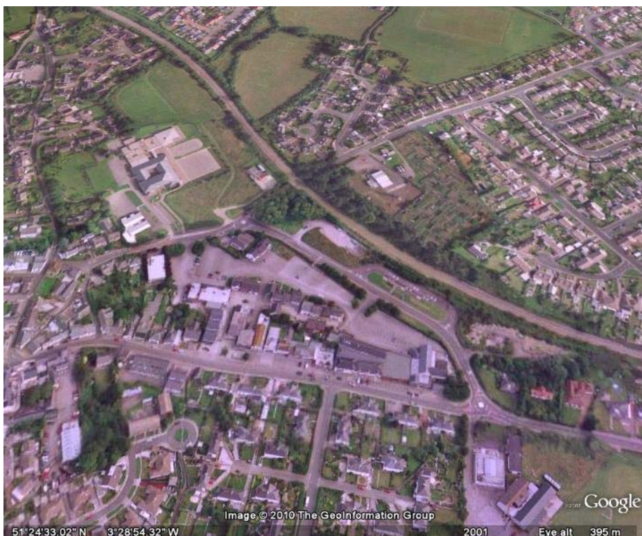
Figure 15 Aerial photograph of Llantwit Major station
