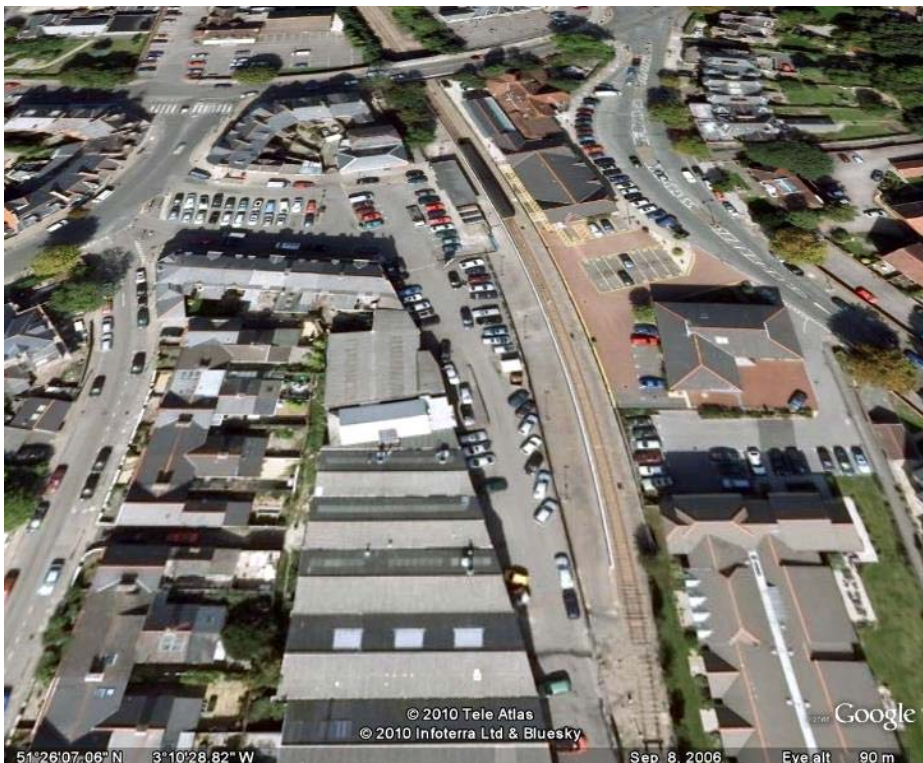
Figure 9 Aerial photograph of Penarth Station
