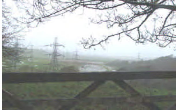
Pylons from Llanberthery to NW
