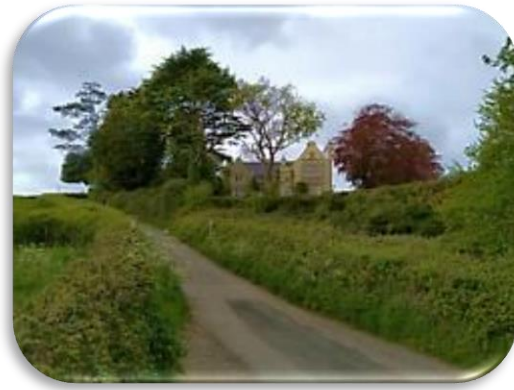
Photograph 7: View of Residential Property from Valley Floor
