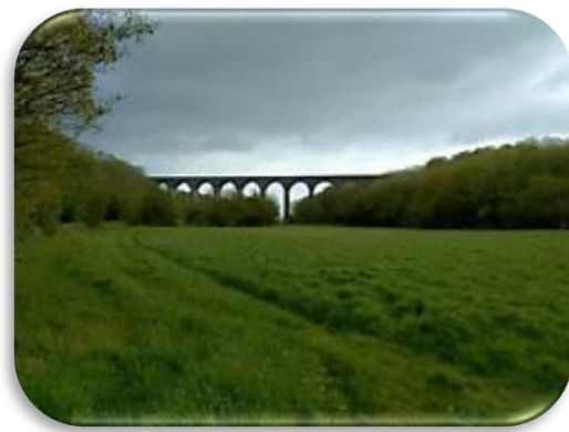
Photograph 8: View of Porthkerry Viaduct from Valley Floor
