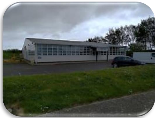
Photograph 5: View of Industrial Unit at Airport (Type 2)
