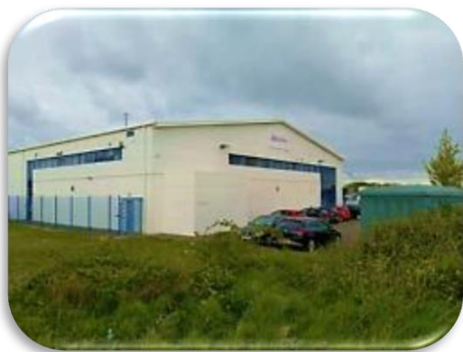
Photograph 4: View of Industrial Unit at Airport (Type 1)
