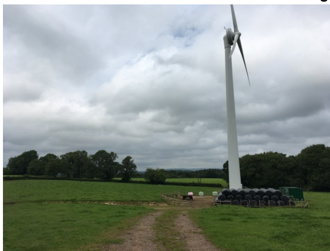
Figure 5: Example of a Medium Sized Turbine in the Vale of Glamorgan
