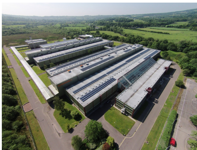
Figure 6: An example of Solar Panels used on Industrial Buildings at the Renishaw Site
