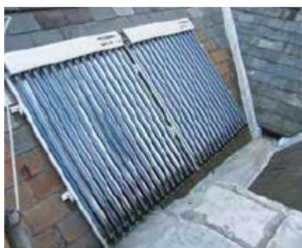
Figure 3: Solar Thermal Collectors Located within Hidden Roof Valley (Source: Cadw)
