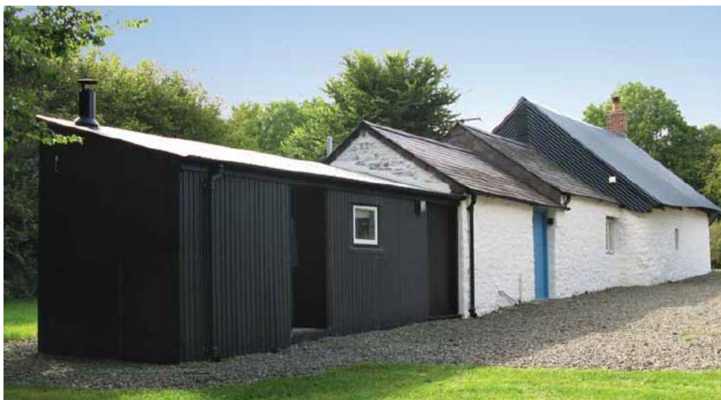
Figure 4: Sensitive Housing of Biomass Boiler in Respect of Listed Building (Source: Cadw)
