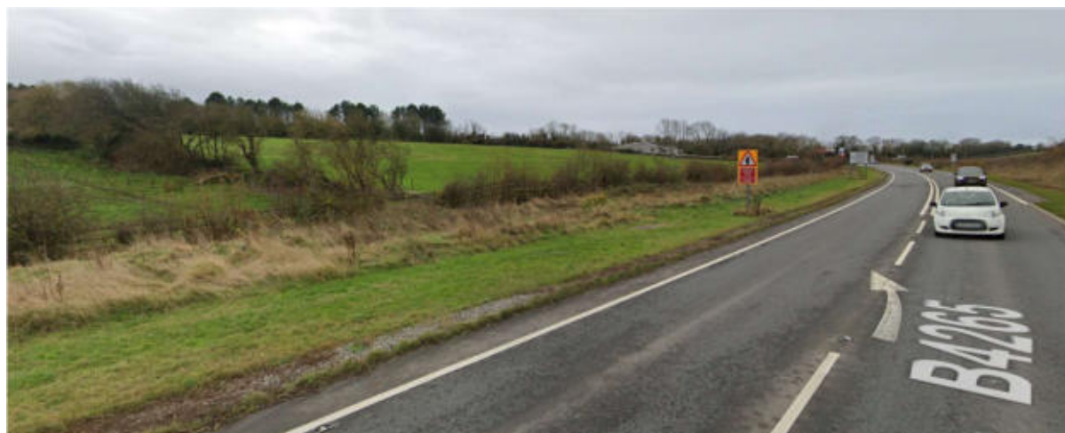
Figure 11 View from B4265 westbound towards Section D 24
