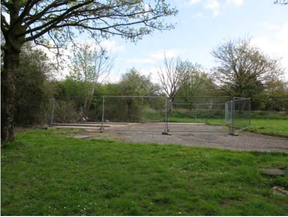
Hard-standing and site of former garages
