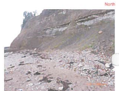
P1 - Debris at base of cliff
