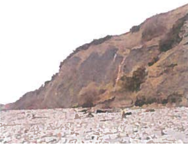
P9 - Faulted area
