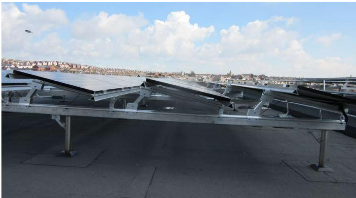
The second Civic Offices 25 kW PV scheme raised the panels off the deck and angled them in order that they would be 'self-cleaning' and be slightly more efficient than the 25 kW system installed on the western roof in 2012. Below the same panels viewed from a southerly elevation.
