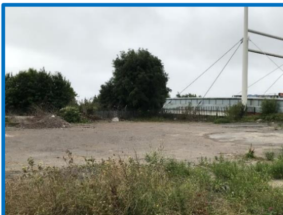
Photo: Gladstone Road Bridge Compound Site
