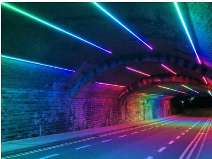
Figure 14: Rail Tunnel Light Improvements
