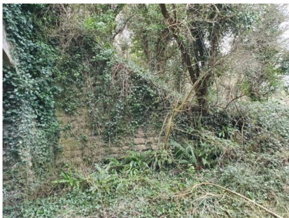
Figure 38 – Additional Structure 3 Wingwall – General Condition
