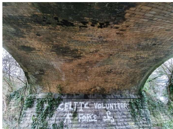
Figure 39 – Additional Structure 3 Arch Barrel
