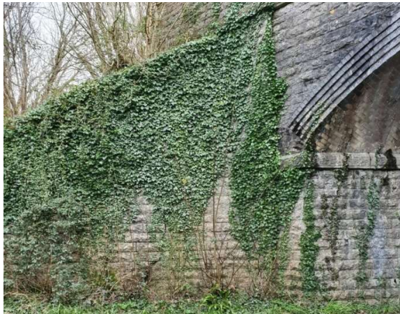
Figure 16 – Fort Road Wingwall – General Condition
