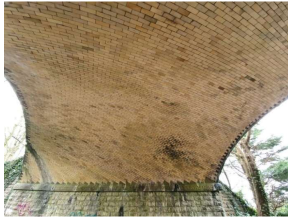
Figure 17 – Fort Road Arch Barrel
