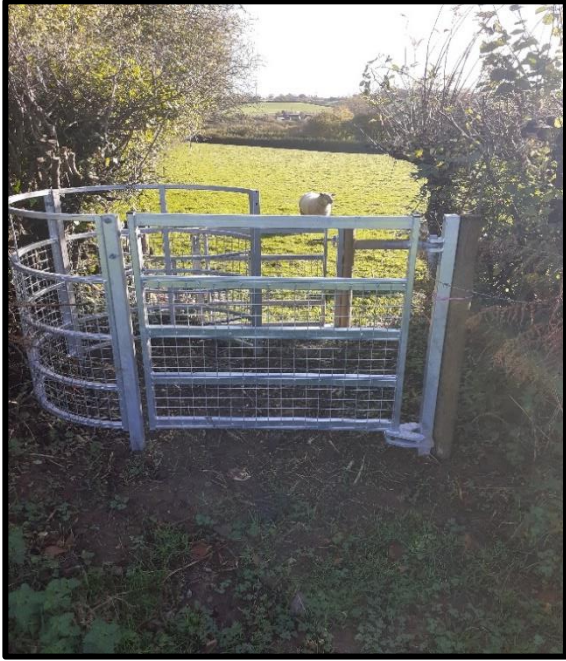
New kissing gates installed – galvanized steel
