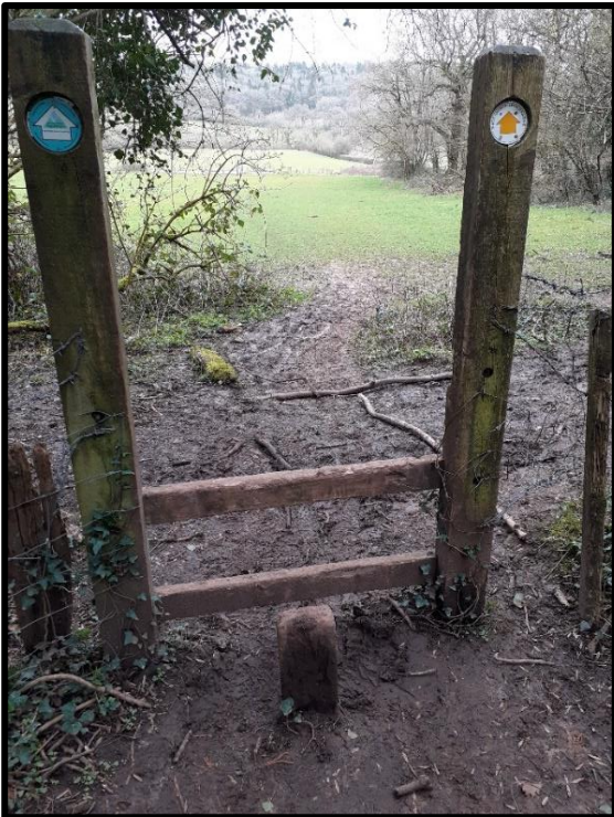
Poor condition of existing stiles - badly deteriorated
