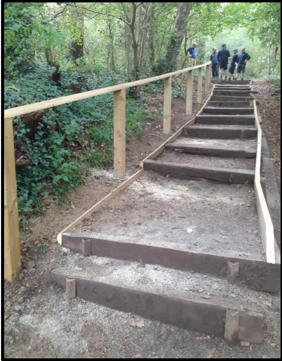
Step and handrail replacements
