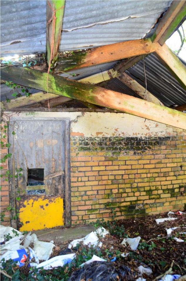
Internal of the building prior to roof being removed, showing roof in a poor and partly collapsed condition (photo supplied by applicant).
