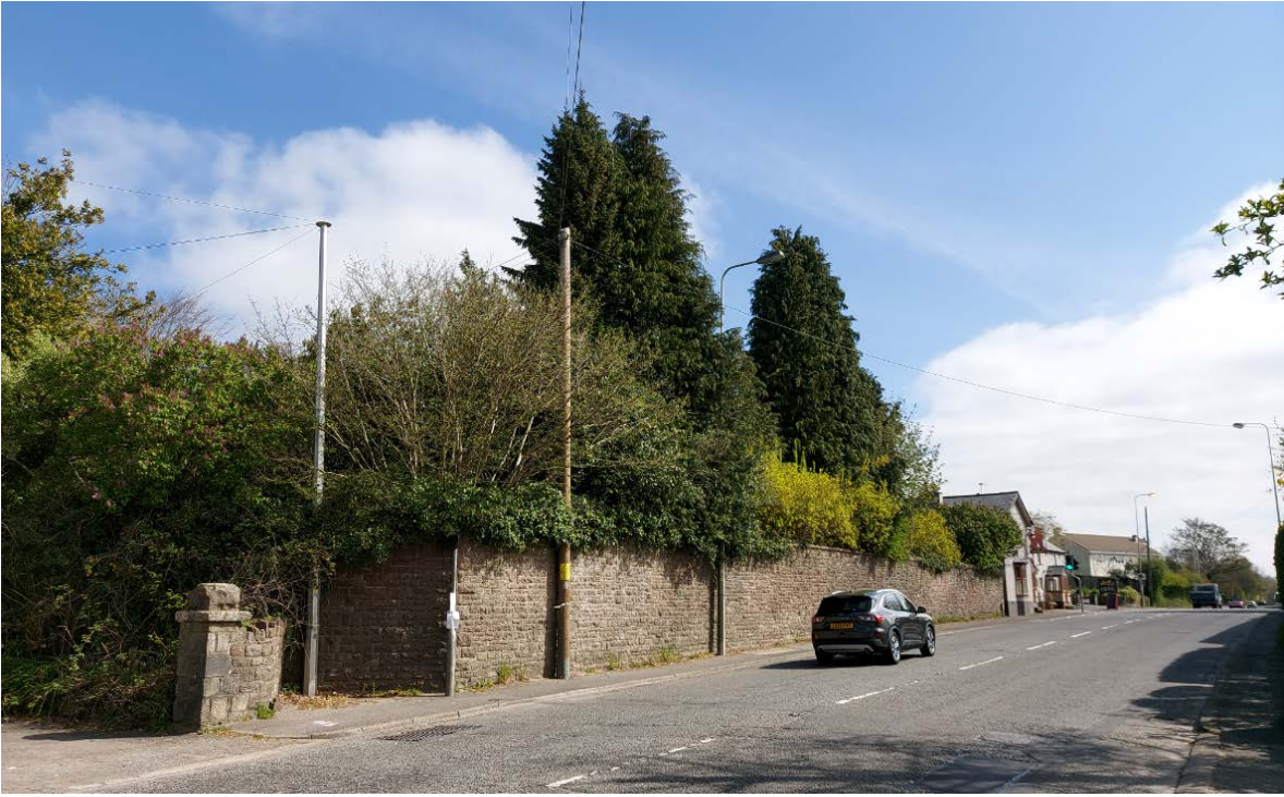
PHOTO OF BOUNDARY WALL
