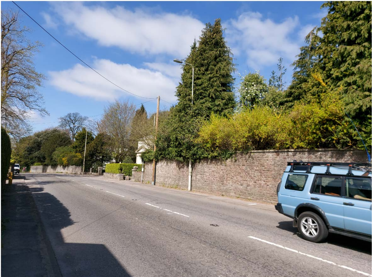
PHOTO OF BOUNDARY WALL
