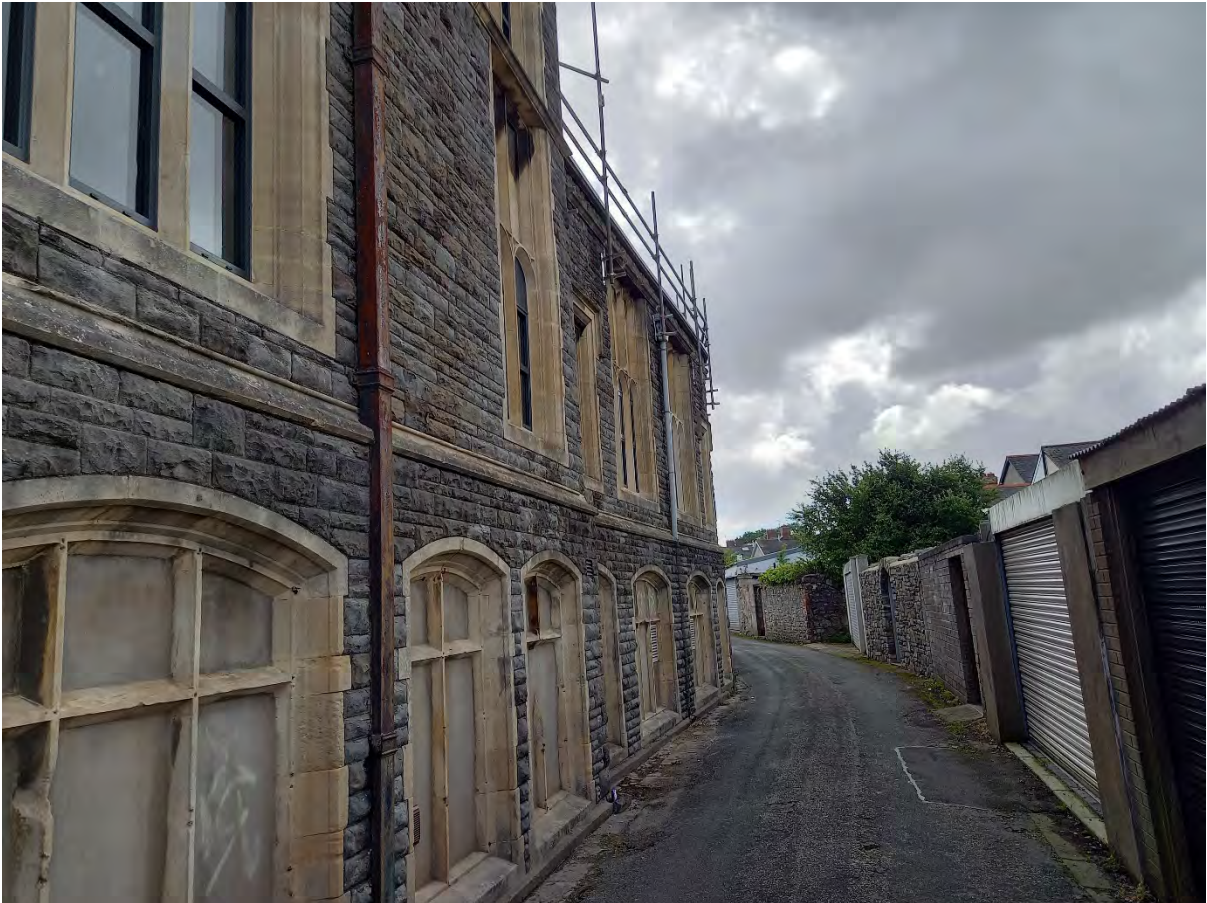
Jubilee Lane showing vents at basement level and boundaries with houses on Clive Place
