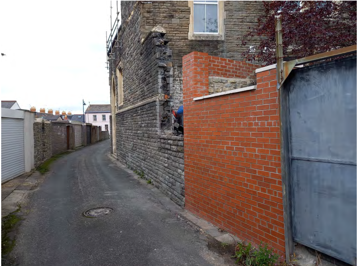
Jubilee Lane and East Elevation showing partially demolished wall and new red brick wall
