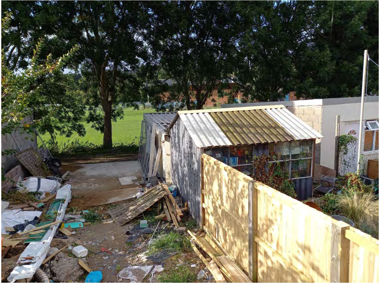
View from inside ground floor window looking towards rear and garden of number 37
