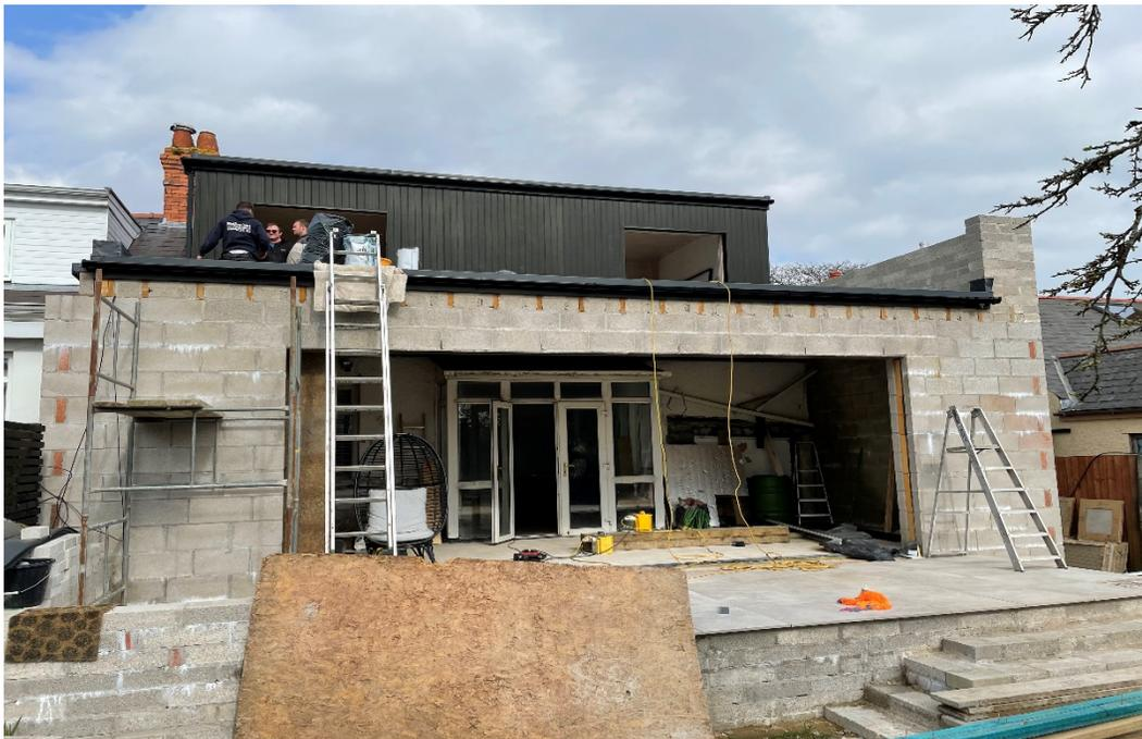
10. During the investigation, it was also identified that the rear extension was being built onto and tied into the external wall of a neighbouring property, with
