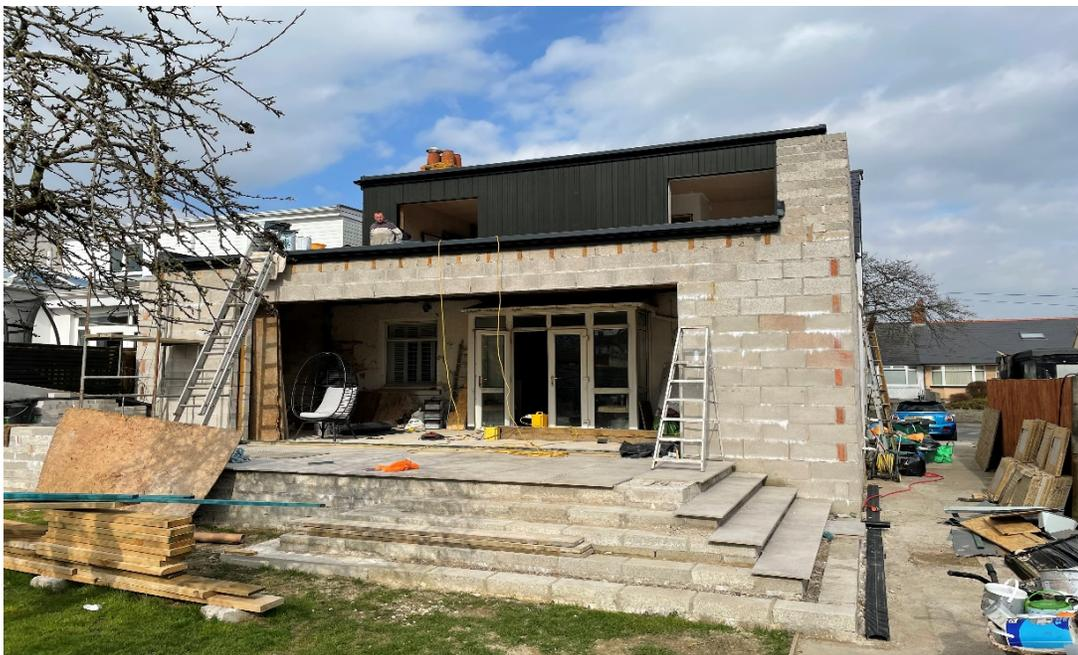
13. During the initial investigation, it was also identified that a raised patio had been constructed to the rear of the extension which runs along the width of the new extension and provides a patio area with steps down into the garden. At a constructed height of 70cm above the existing ground level, this exceeds the PD rights for raised patios which is 30cm and therefore requires planning
