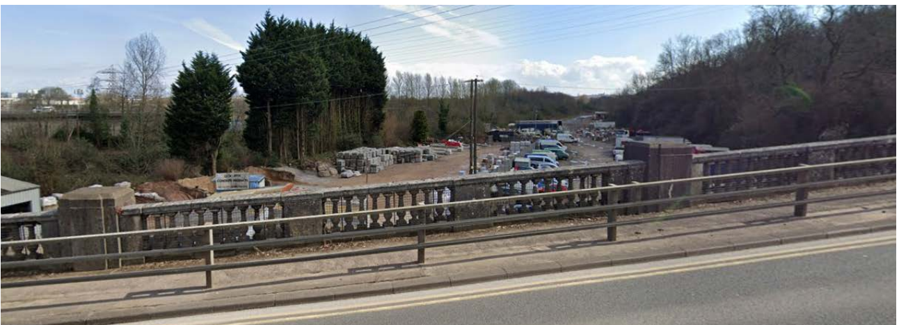
View towards northern section of site from viaduct
