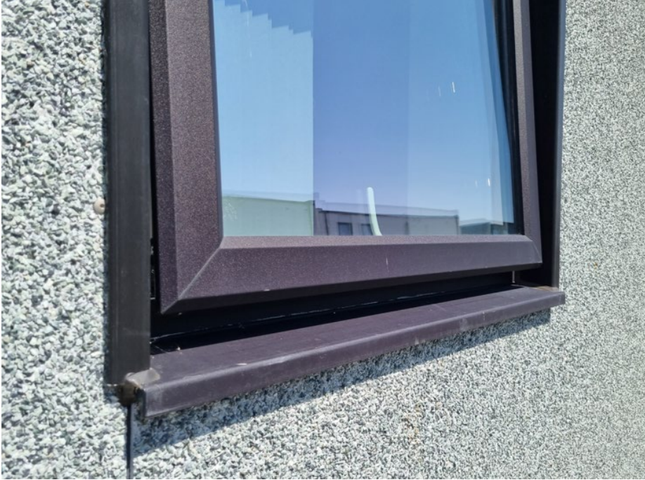
Fig 6: Photo of window with quick release restrictor engaged
