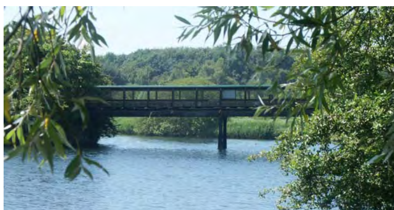
Mile Road Bridge spanning West and East lakes at Cosmeston
