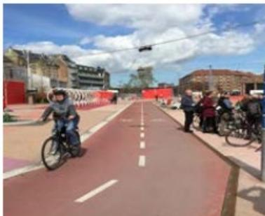
**Separation of pedestrians from cyclists and motor traffic through provision of segregated off-carriageway infrastructure; if necessary through reallocation of road space**
