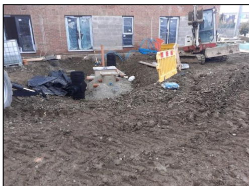
Rainwater harvesting system installed at Llon Yr Ysgol – during and after installation.
