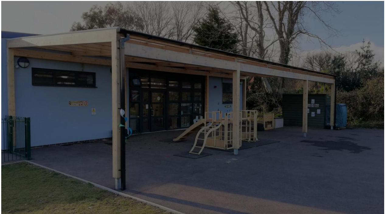
Figure 2: Image of St Josephs Primary School building (outside view)
