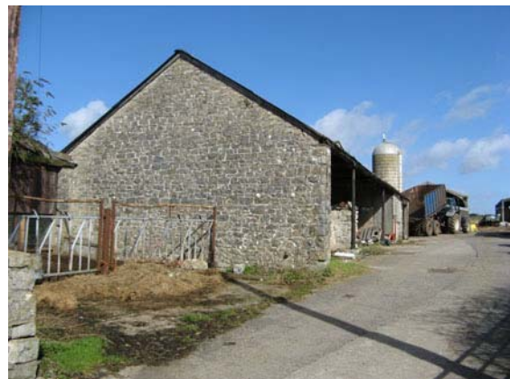
Local lias limestone is the prevalent building material, especially of farm buildings.
