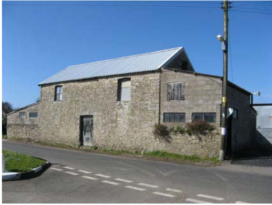
Farm buildings are a feature of the village.
